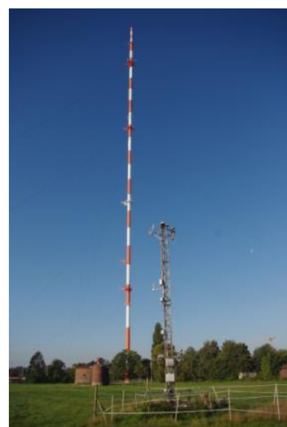
The “Wettermast Hamburg” site. Measurements of the lower tower (right) are used.
